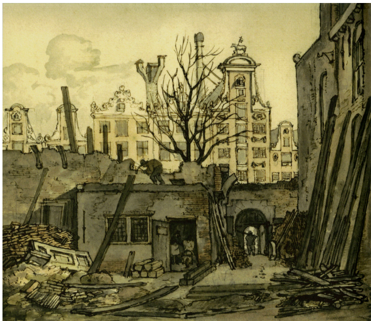
The demolition of the West Indian House on the Singel in Amsterdam, Gerrit Lamberts, 1817, Collection Van Seghen, Stadsarchief, Amsterdam, in den Heijer, Geschiedenis van de WIC , p. 186.
