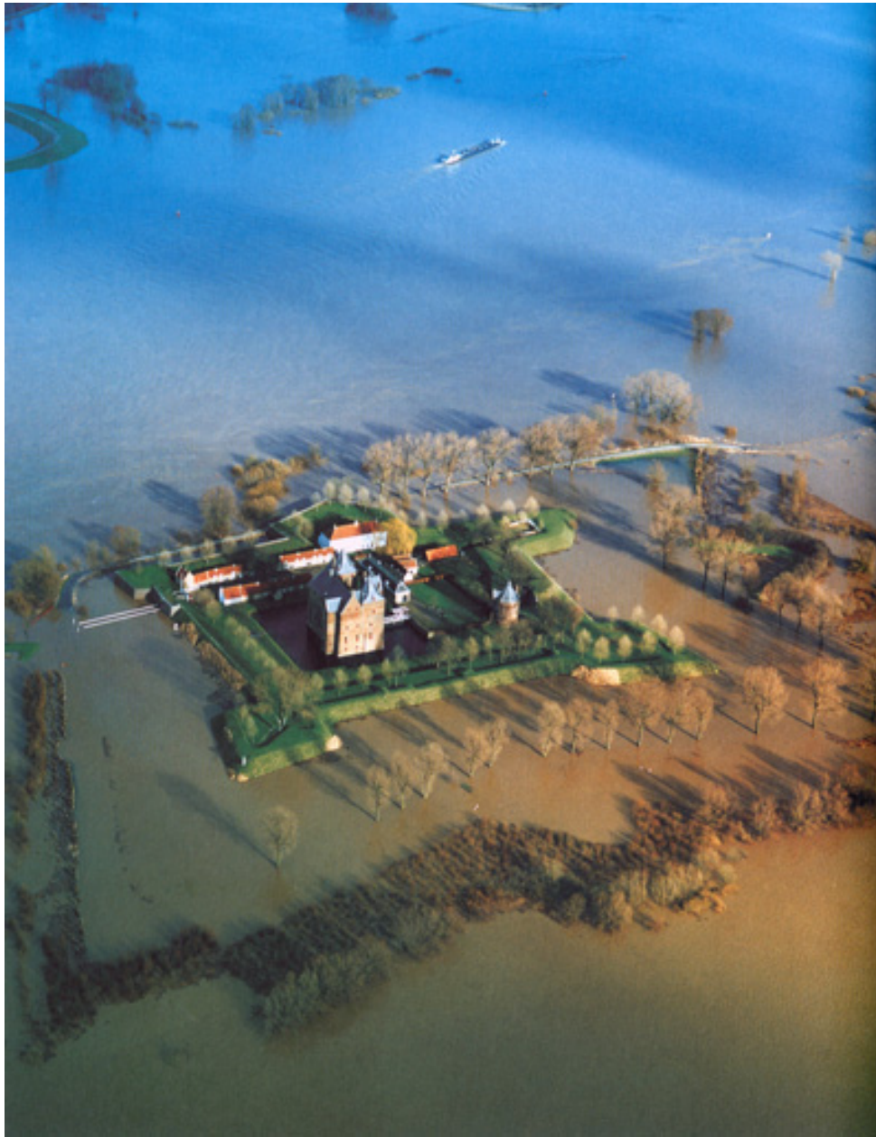
An aerial view of Slot Loevestein, a 14 th century water castle, during extremely high water in 1995. The earthen walls with bastions were built during the 16 th and 17 th centuries and are visible in the muddy water, Will, Sterk Water , p. 8.
