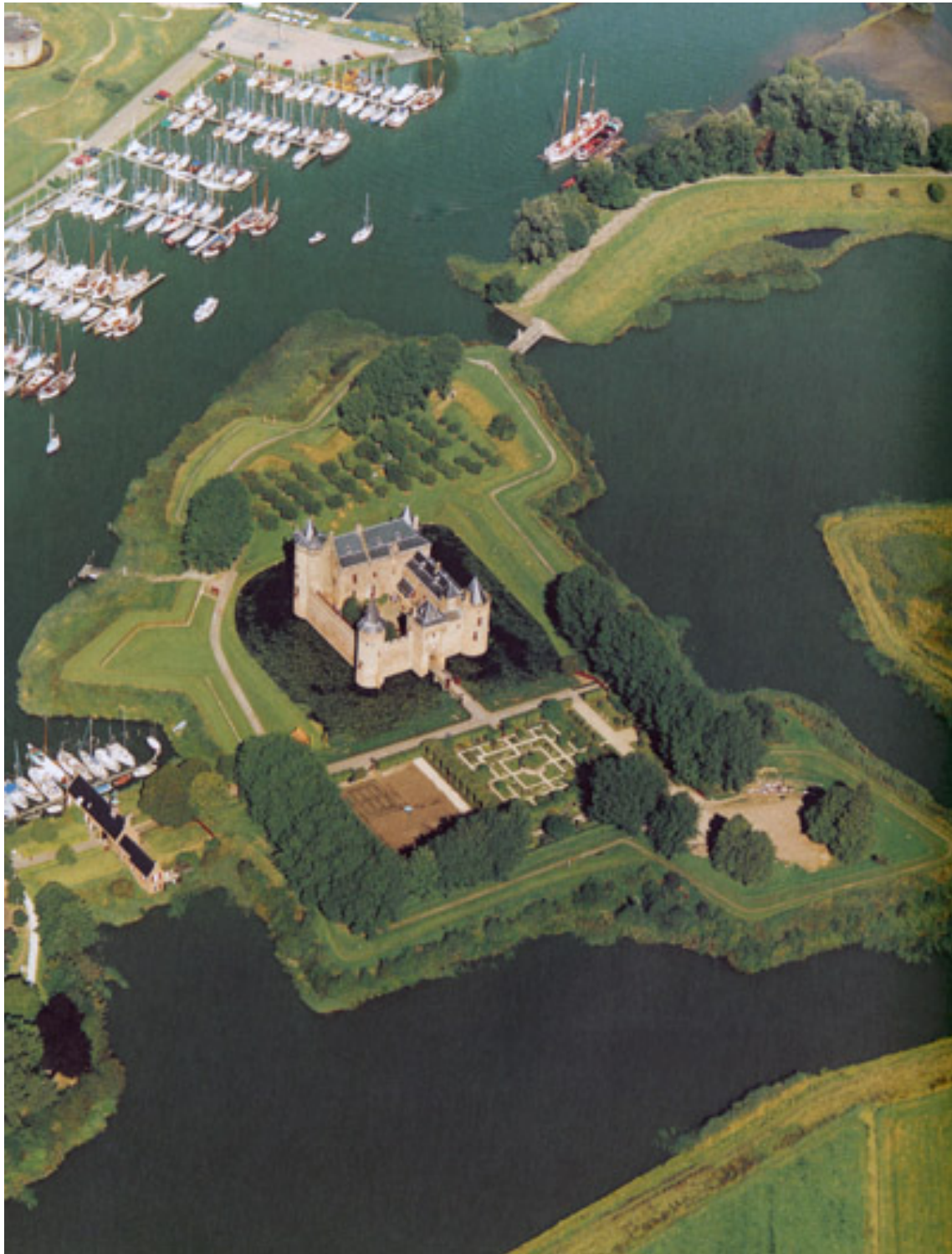
Muiden Castle at the mouth of the Vecht with its 18 th and 19 th century earthen walls protected the northern end of the Utrechtse waterlinie at Vecht, Will, Sterk Water , p. 28.
