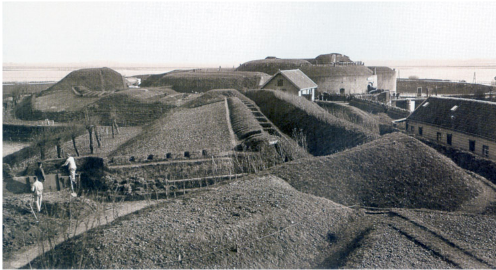
Fort Vuren on the Waal. Originally built in 1864, it was rebuilt during the 1870s. Photo of 1915, Will, Sterk Water , p. 64.
