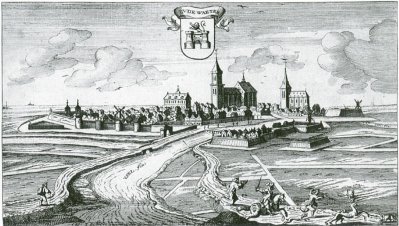
The fortified city of Oudewater was included in the waterlinie in 1673. The print still shows the medieval city walls. The new bastions on the right protected the city. Will, Sterk Water , p. 41.
