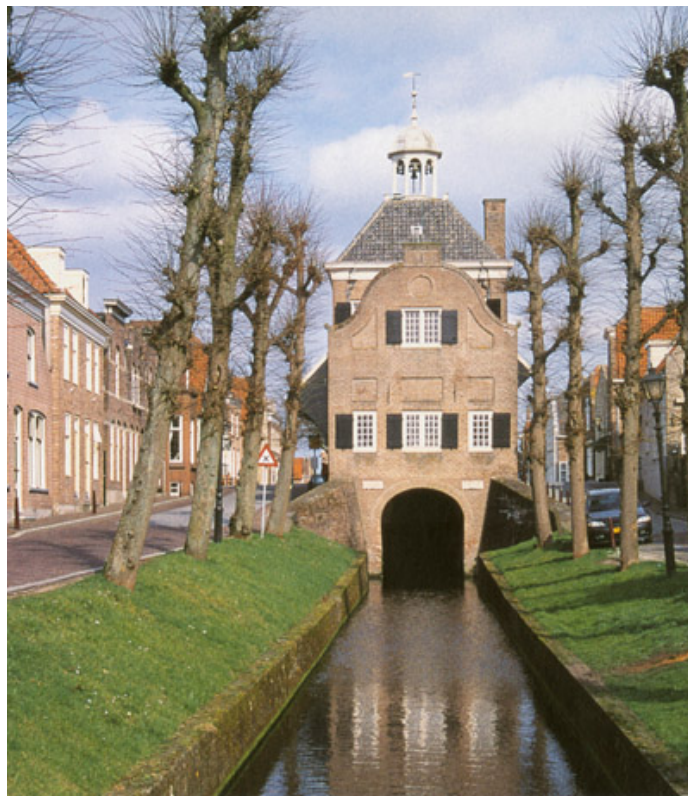
The canal used for inundation is situated underneath the Town Hall of Nieuwpoort in the middle of town to protect it from sabotage from the farmers, Will, Sterk Water , p. 47.
